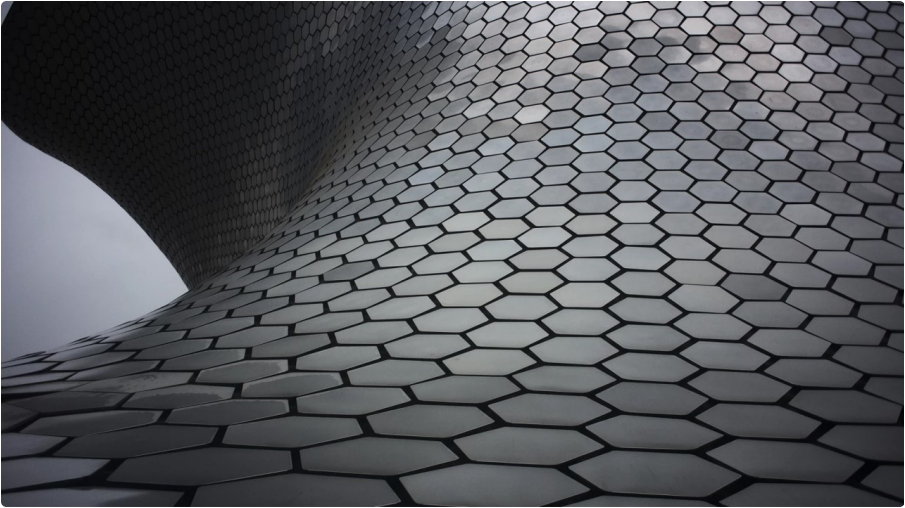
Figure 11.1. Soumaya Museum, Mexico City. Its facade required model-based fabrication coordination of 14,808 unique panels. Image: construbim.com.
